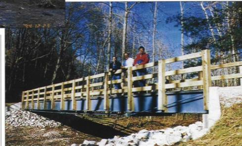
pultruded composite I-beams (glass-fiber-reinforced vinyl ester with carbon fiber in the flanges to increase stiffness).
